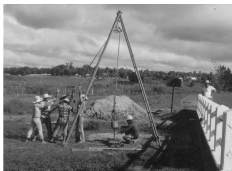
Figura 2. Ensayo del Standard Penetration Test.
